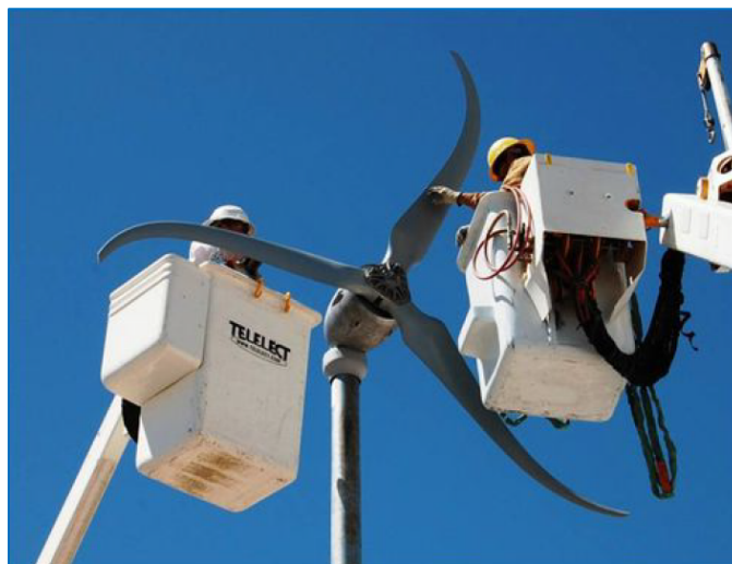
Figure 6. Maintenance of a Wind Turbine
