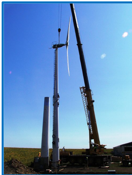
Figure 7. Installation of a Wind Turbine
